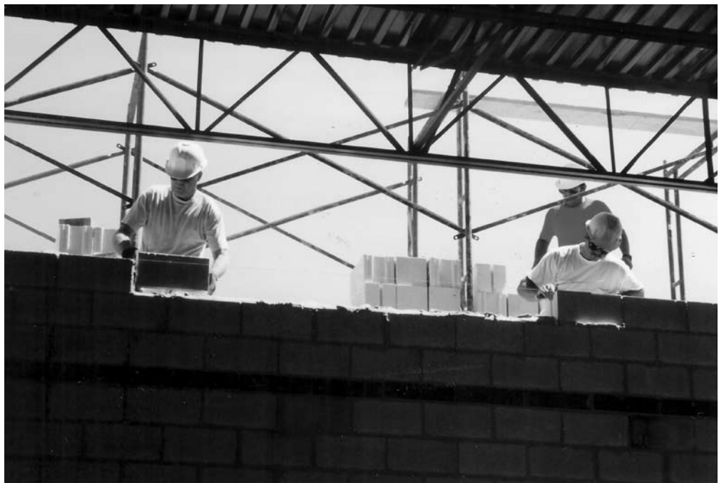
Placement of Concrete Masonry Units
