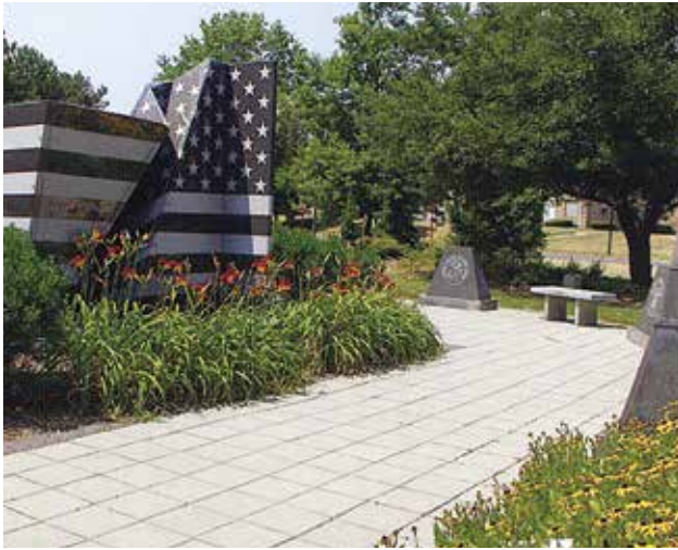
Figure 14. High SR paving slabs
