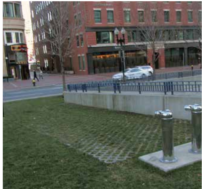
Figure 13. Concrete grid pavement typically reduces runoff in a manner similar to grassed surfaces and are best used to earn heat island reduction points.
