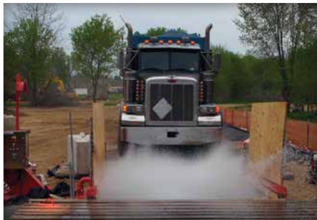
Figure 11. Larger PICP projects may require tire washing equipment for trucks to keep mud from contaminating PICP aggregates.
