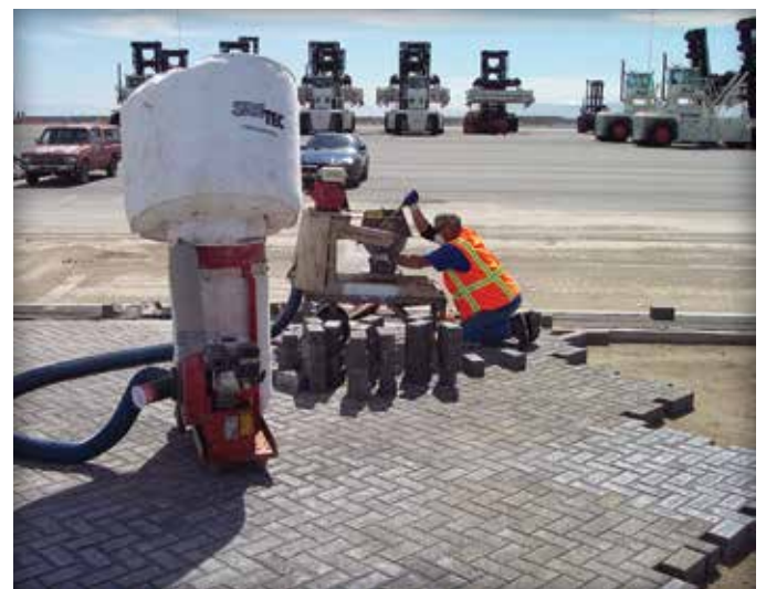
Figure 8. Saw cutting pavers.
