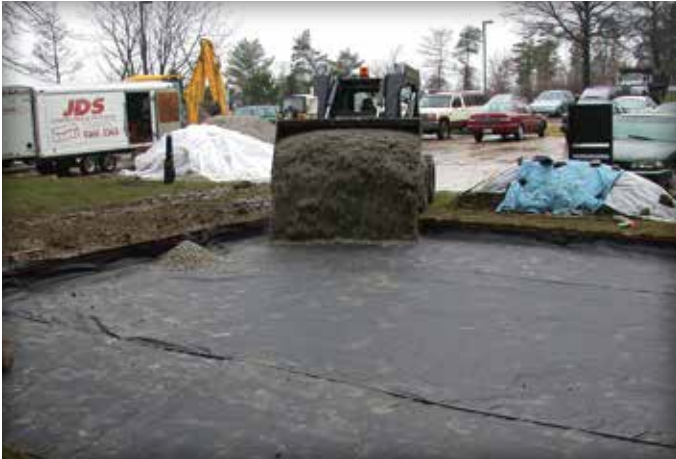
Figure 3. Application of the geotextile under aggregate base.
