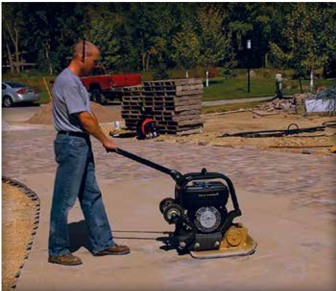
Figure 11. Vibrating sand into the joints.
