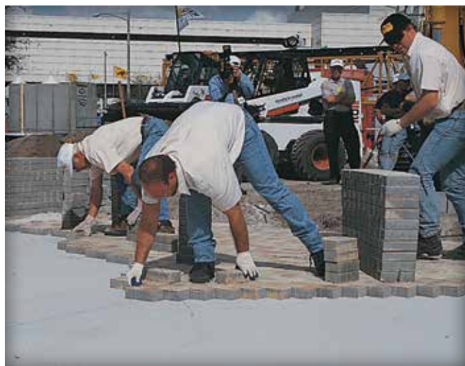
Figure 7. Placing the concrete pavers.
