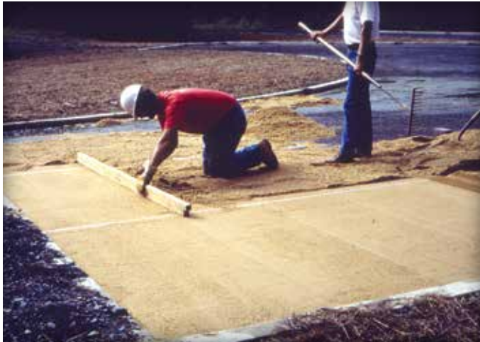
Figure 6a & 6b. Screeding the bedding sand.
