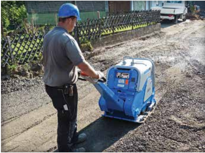
Figure 4. Base compaction with a reversible plate compactor.
