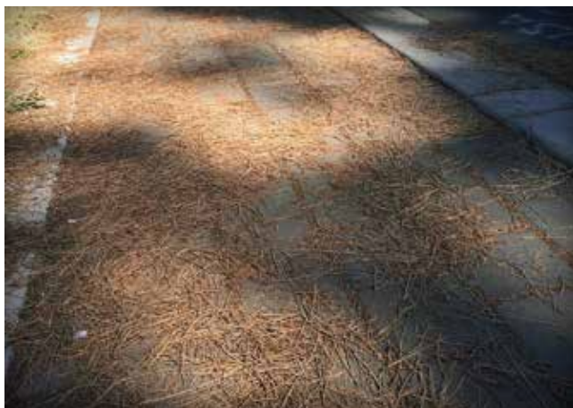
Figures 7 and 8. Pine needles and leaves eventually will degrade and get compacted into the joints from traffic. They should be removed by sweeping or vacuuming before that happens.
