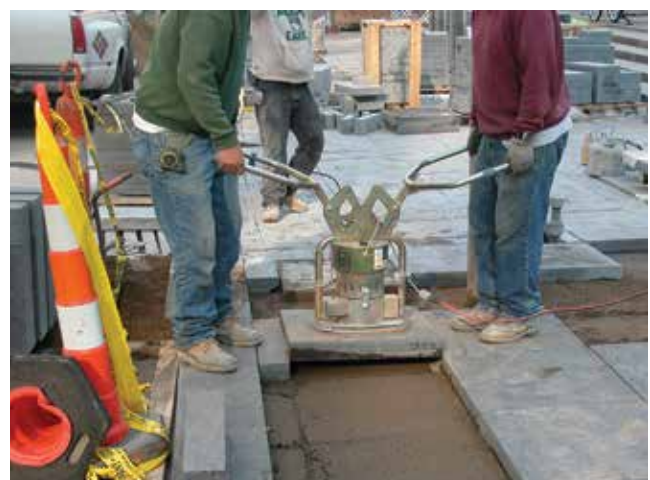
Figure 14. Two-person vacuum lift for larger paving slabs.
