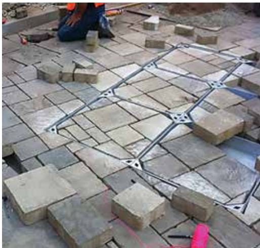
Figure 27. Another example of cutting pavers to accommodate a utility cover set at an acute angle to the paving slab pattern
