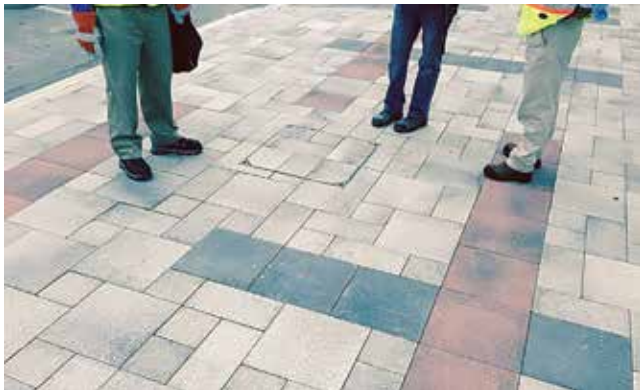
Figure 26. Example of a utility cover that does not fit neatly into the paving pattern.
