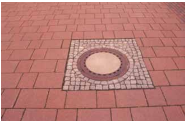
Figure 28. Filling the outside of a utility cover with mortar-set stone paving units
