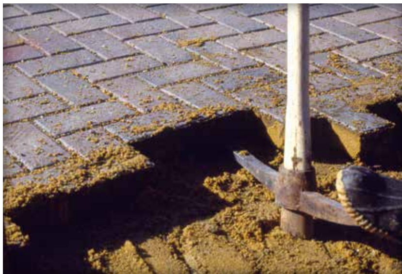
Figure 6. Prying out the remaining pavers
