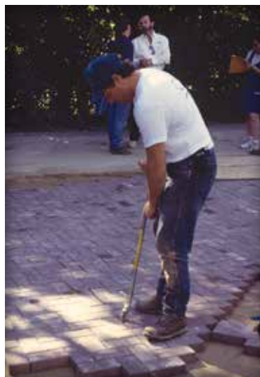
Figure 13. Adjusting joint spacing and alignment.
