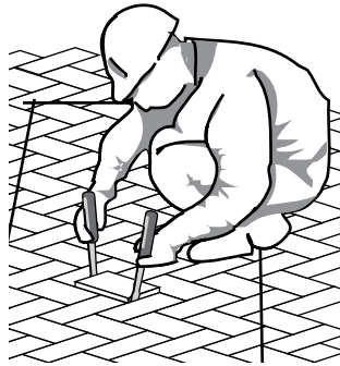
Figure 3. Prying the paver upwards with two large screwdrivers.
