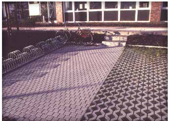
Figure 14. Solid pavers used for bicycle parking and pedestrian access.
