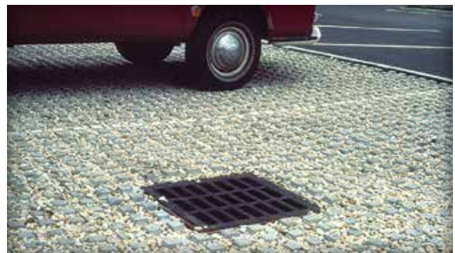
Figure 16. Concrete grids with aggregate in the openings
