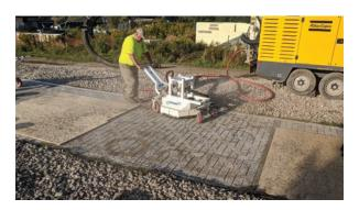
There is an ongoing study through the University of Toronto and NSERC that is investigating maintenance best management practices for PICP. New and innovative maintenance equipment, like the Typhoon PICP Joint Cleaning system are being introduced and evaluated. Contact Oaks for updates and information on the test results.
