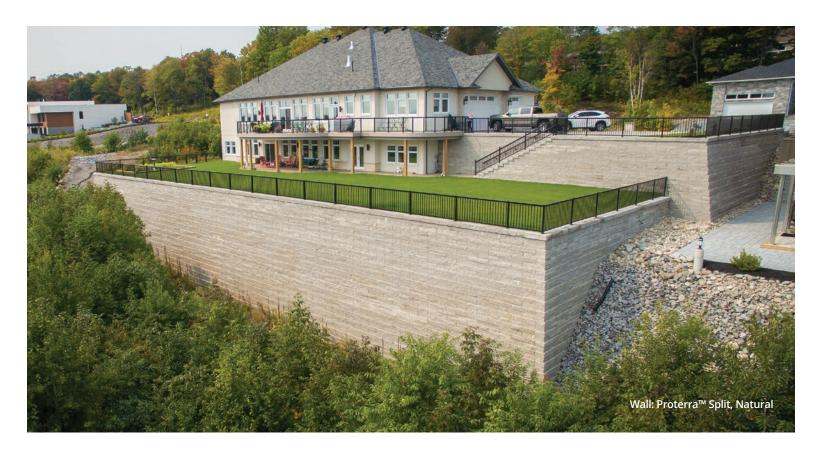
Retaining walls are commonly used to create more usable space onsite, particularly where there are dramatic grade changes over short distances. The rear yard in the above photo would have been un-usable by the home owner without the addition of the retaining walls, and accessibility is maintained between levels through built in staircases.
