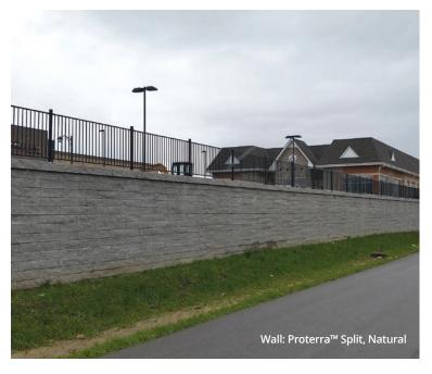
In commercial applications, consideration must to be given to providing easy access to customers/clients. A retaining wall was used in the adjacent project to "flatten" the parking lot making it easier to push around the available shopping carts.
