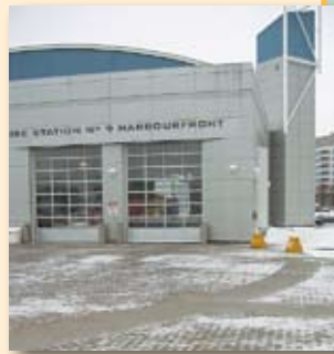
PICP withstands salt and snow plowing, a regular part of Toronto winters.
