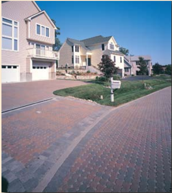
Runoff quantity and quality from driveways were monitored from water exiting slot drains.
