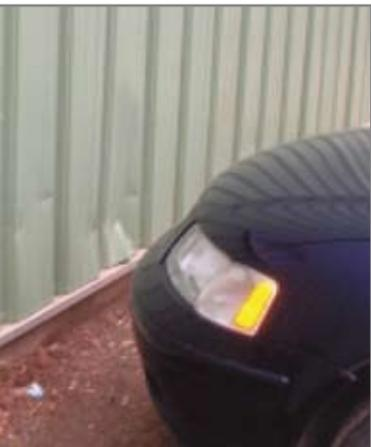
*Steel cladding dented by parking cars.*
