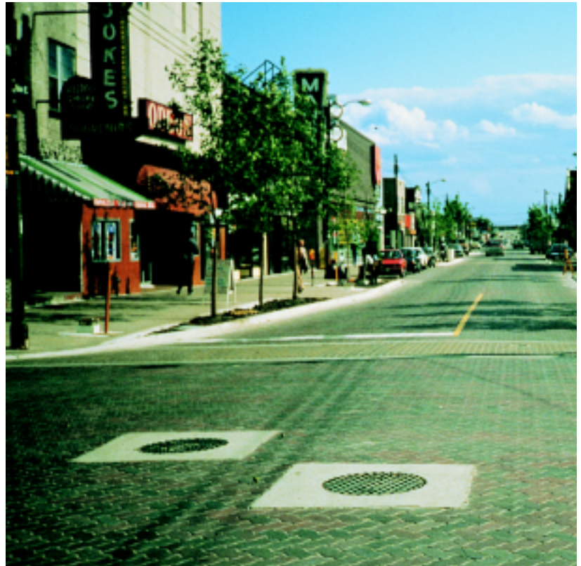
Figure 7. Concrete collars protect utility structures.
