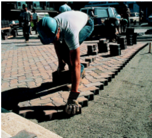
Figure 8. A herringbone pattern in the street provided resistance to turning,
