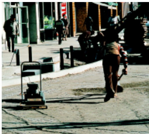
Figure 11. Sand swept into the joints and compaction of the pavers transform the pavement from a loose collection of units to an interlocking load-bearing pavement system.
