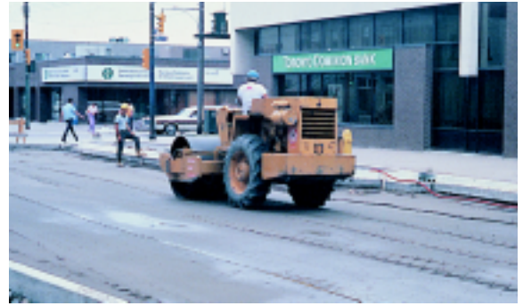
Figure 5. Compaction of the base is essential to all flexible pavements including those built with concrete pavers.
