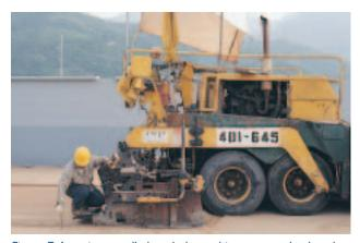
Figure 7.A sonic-controlled asphalt machine accurately placed, <sup>3</sup>/<sub>4</sub> in. (20 mm) thick bedding sand layer over a smooth CTB surface.
