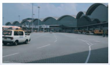
Figure 2. Interlocking concrete pavements were selected because they would tolerate expected settlement around the terminal building and remain serviceable.
