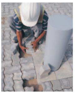
Figure 13. Cut pavers were fitted around concrete collars at bollards and at utility structures.
