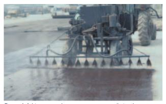
Figure 6.A bitumen tack coat secures geotextile in place over the CTB. A thin layer of sand was then spread to keep the bituminous material from sticking to boots and tires.
