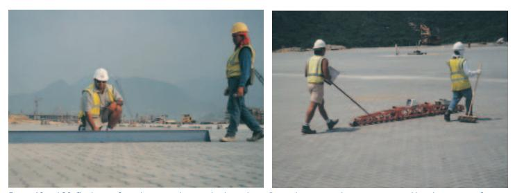
Figures 19 and 20. Checking surface tolerances with a straightedge and overall smoothness ensured a pavement amenable to keeping aircraft level during refueling.
