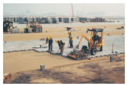
Figure 10. Mechanized installation accelerated paving by using three machines to place layers of pavers in their final herringbone laying pattern. Note the bundles of pavers in the background and the crew adjusting joint lines and tightening each layer against its neighbors.
