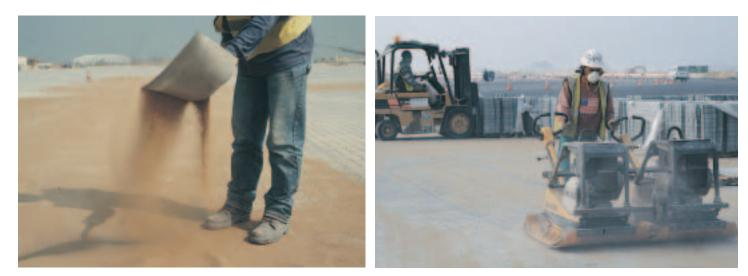
Figures 16 and 17. Dry joint was distributed across the compacted pavers and compacted into the joints until full. The joint sand gradation was finer than the bedding sand.
