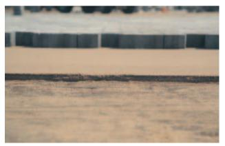
Figure 8. The screeded bedding sand maintained a consistent thickness since the surface of the CTB met tolerances for smoothness.
