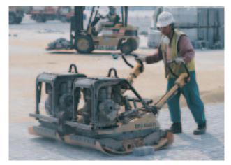
Figure 15. 9,000 lbf (40 kN) plate compactors were used to compact the pavers into the bedding sand, then again to compact the joint sand into the joints. Two were joined for greater efficiency.
