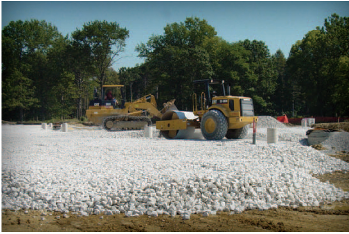
Base and Subbase construction for parking lot
