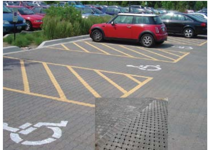
Figure 7. PICP combined with solid interlocking concrete pavers accommodates accessible parking and pedestrian areas.
