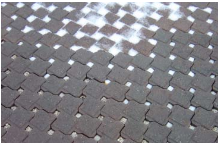
Figure 8. PICP surface openings promote faster snow melting thereby reducing hazardous ice in winter.
