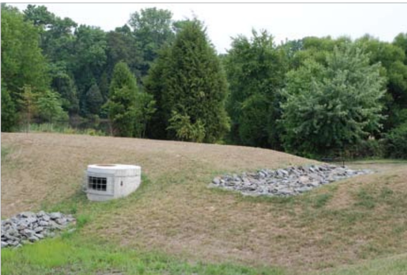
Figure 1. On-site infiltration practices such as permeable pavement are emerging as preferred stormwater management solutions to off-site controls that consume valuable land including detention (foreground) and retention (background) ponds shown here. Permeable pavement can reduce or eliminate these facilities.
