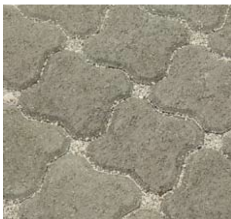
Figure 3. Left to right: After excavation, PICP construction begins with placing and compacting an open-graded subbase and base as shown in the first two photos. The next photo shows mechanical installation of the concrete pavers on a screeded bedding layer of small aggregate. The rightmost photo illustrates small aggregate in the openings and joints that enable high surface infiltration. The pavers and aggregate are compacted to create and interlocking pavement.
