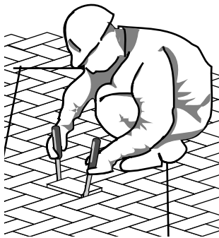
Figure 3. Prying the paver upwards with two large screwdrivers.
