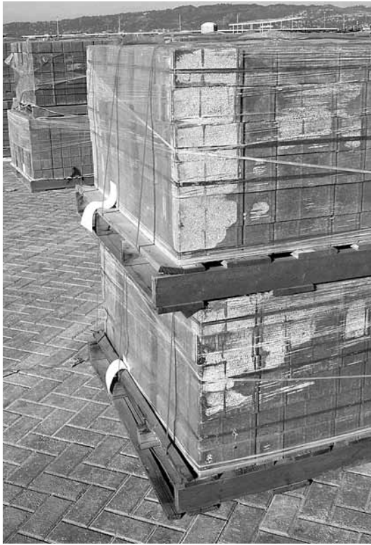
Figure 2. Bundles of ready-to-install pavers for setting by mechanical equipment. Bundles are often called cubes of pavers.
