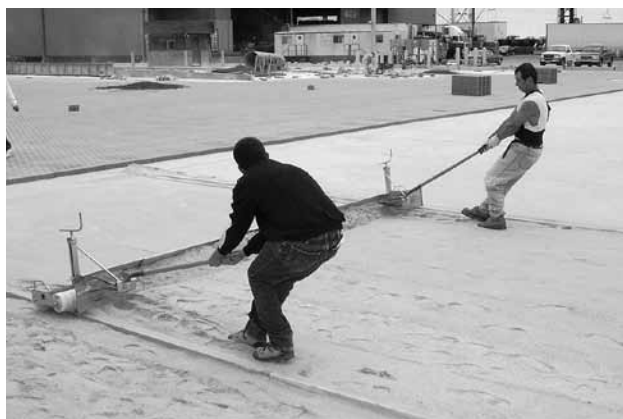
Figure 4. A two-man hand pulled screed
