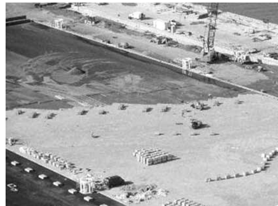
Figure 7. Maintaining an angular laying face that resembles a saw-tooth pattern facilitates installation of paver clusters.
