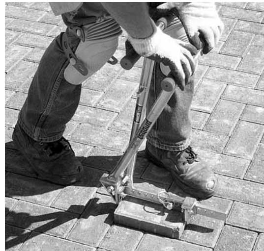
Figure 10. During initial compaction, cracked pavers are removed and immediately replaced with whole units.
