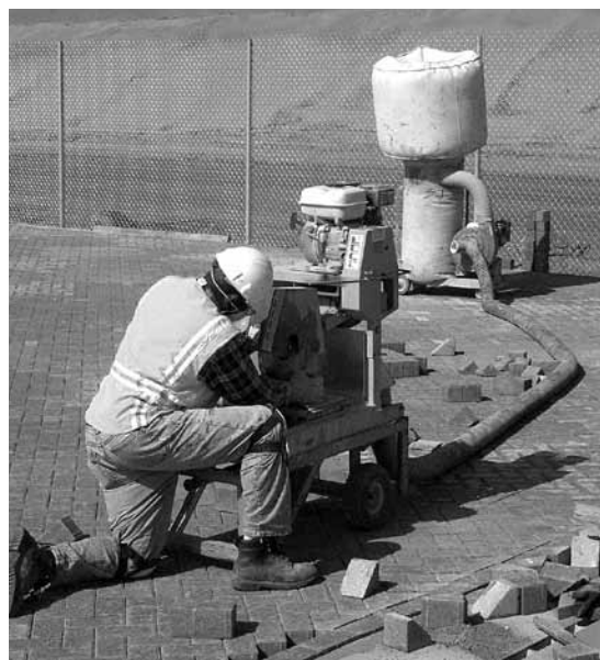
Figure 8. Edge pavers are saw cut to fit against a drainage inlet.
