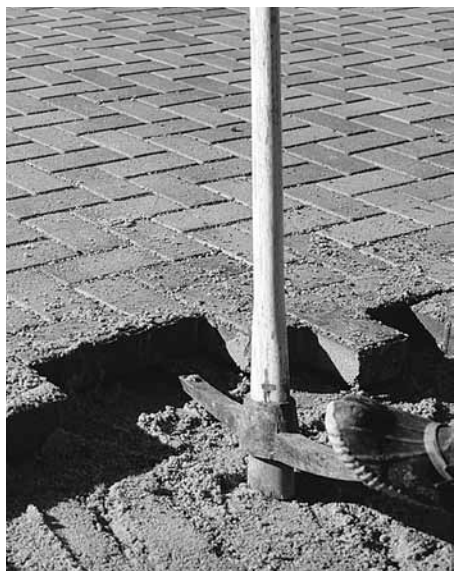
Figure 6. Prying out the remaining pavers
