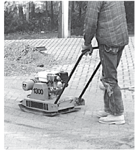
Figure 13 (Left). Adjusting joint spacing and alignment. Figure 14 (Right). Second and final compaction of the pavers. The first compaction occurs after the pavers are placed (no sand in the joints). The second compaction works the sand on pavers into the joints. This process causes the pavers to interlock.
