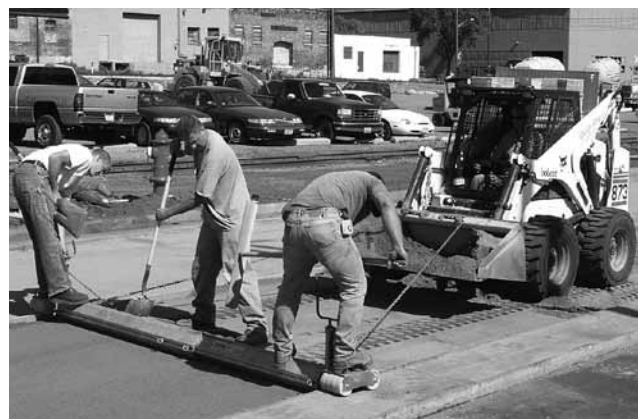
Figure 5. Mechanical screeding is the most efficient method of bedding sand installation
